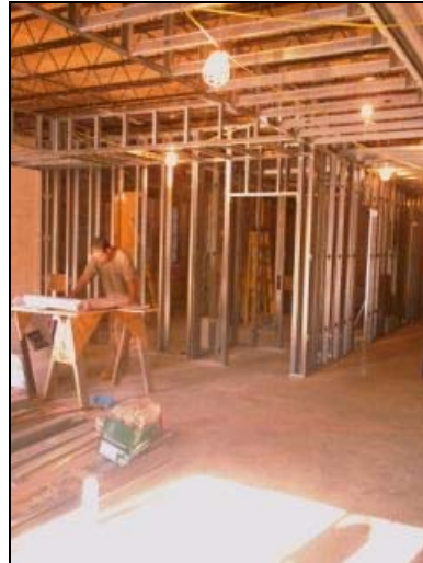
Framing in the library
