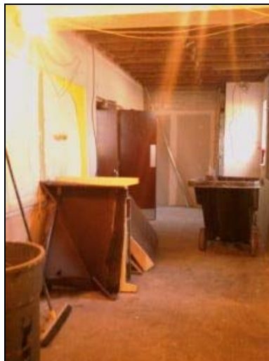
Hallway outside the church office
